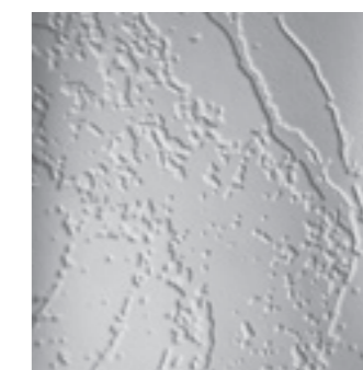
Concrete Wall - WP30004TX45
